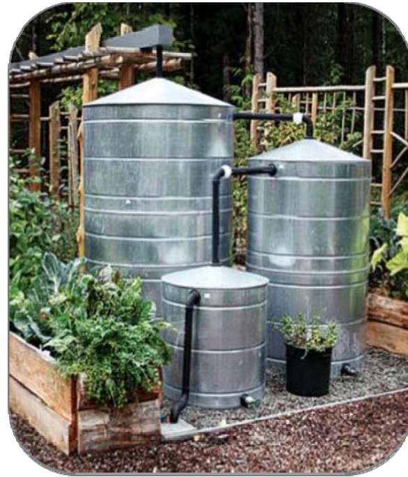
Daisy chained system of metal barrels Courtesy of Sunset Magazine
